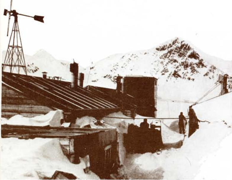
Harnessing wind throughout the world, Wincharger installations like this one in Iceland brought electricity to remote areas.
