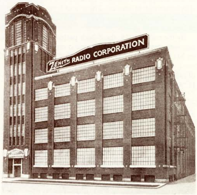
In 1924, burgeoning Zenith moved to this factory at 3620 Iron Street.
