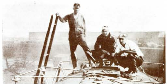
Zenith equipped the first train to use short wave radio. Above is the New York Central antenna installation. G. E. Gustafson (left), the young engineer who built and installed the equipment, has been chief engineer since 1934 and vice president in charge of engineering since 1943. Below is view of caboose before test run.
